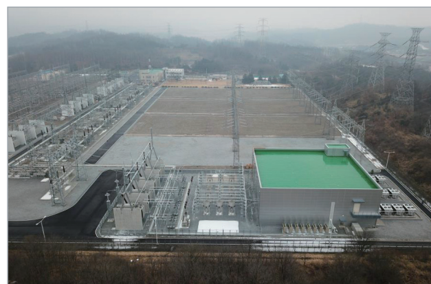
[Fig. 2] New \pm 400\text{Mvar} STATCOM in Yeongju
