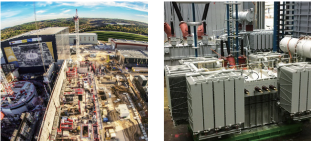
[Fig. 7] View of the ester oil transformers supplied by Hyosung to ITER (International Thermonuclear Experimental Reactor) in France and a refinery plant in Oman
