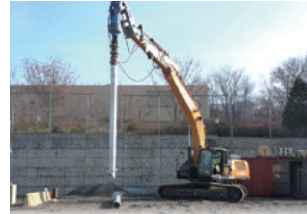
A machine driving helical pile into the ground
