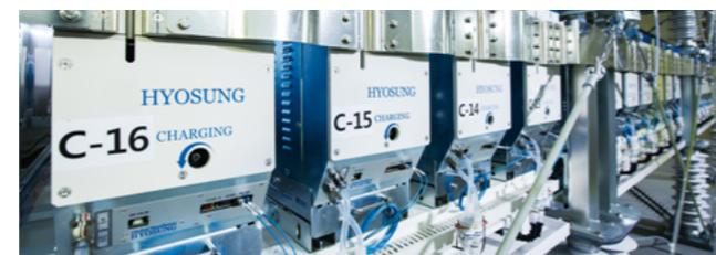
Static Synchronous Compensation (STATCOM) by Hyosung Heavy Industries
