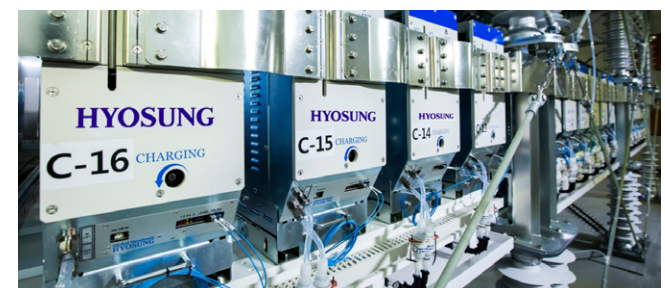
Static Synchronous Compensation (STATCOM) by Hyosung Heavy Industries
