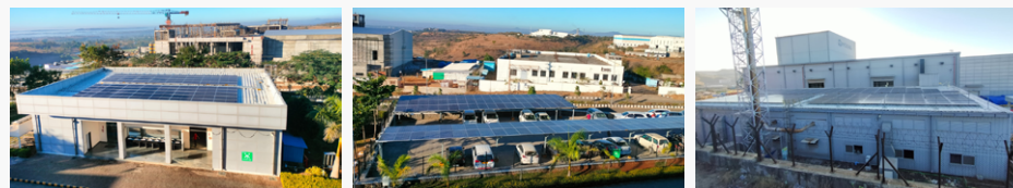
Canteen Roof Solar
