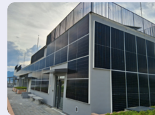
Installation of solar panels on roofs and exterior walls of apartment complexes
